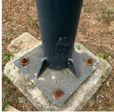
Figure 2: Streetlight pole base
