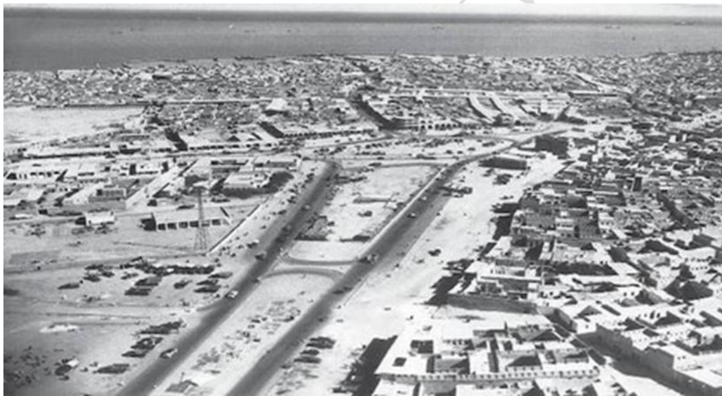
Figure 2: Old City of Kuwait Redevelopment After the Discovery of Oil
