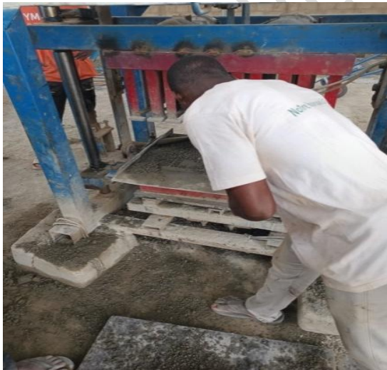
Figure 4.a: Pouring the mortar into the mould
