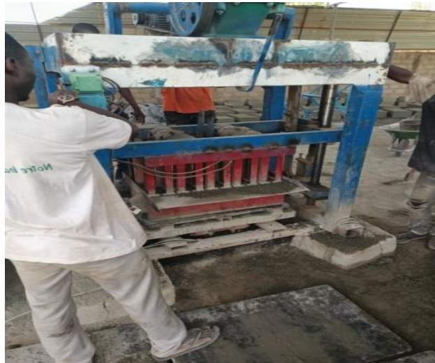
Figure 4.b: Compaction of mortar
