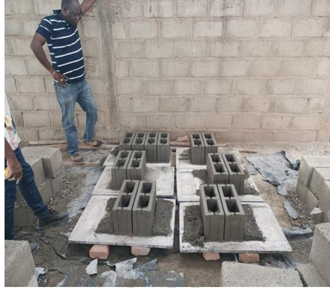
Figure 4.d: Storage of concrete blocks
