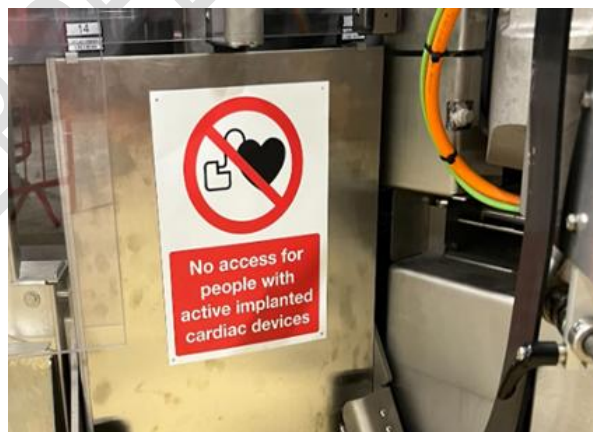
401 402 Figure 3. Safety Signage
