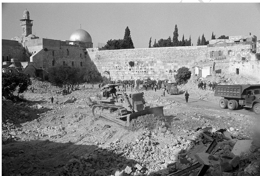
Figure 1. Demolition of the Mughrabi Quarter
